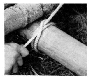
Make a pigtail of the running and standing ends of the rope similar to a timber hitch, and pull it snugly over the first spar of the floor.
