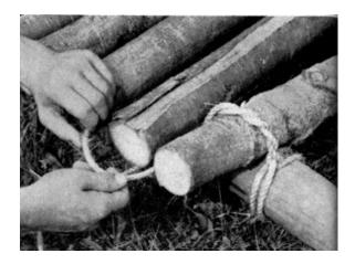
Then pull a bight under the support timber, and up between the first two spars. Then slip the bight over the end of the first spar.
