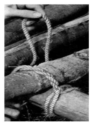
Now pull the rope under the support timber and up over the second spar on the outside of the timber. Then repeat each step, alternating pulling the bight from the inner side of the support timber to the outer side of the timber, lashing each successive spar to the bottom support timber.
